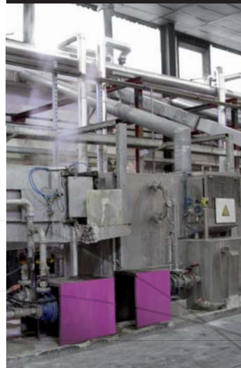
3 Degreasing and rinsing
